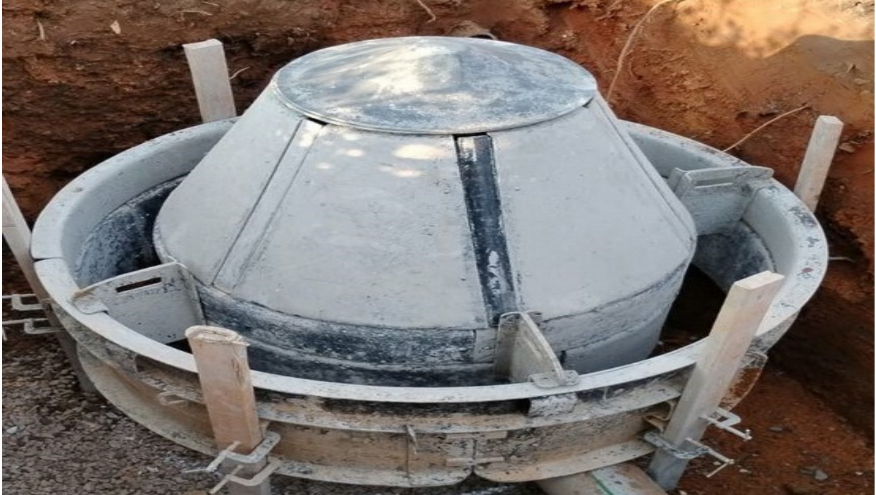
CAST-IN-PLACE MANHOLE CONSTRUCTION PROCESS
