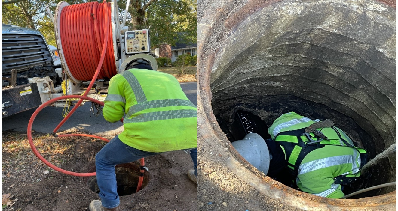
PRE-REPLACEMENT CLEANING WORK IN SANITARY SEWER LINE
