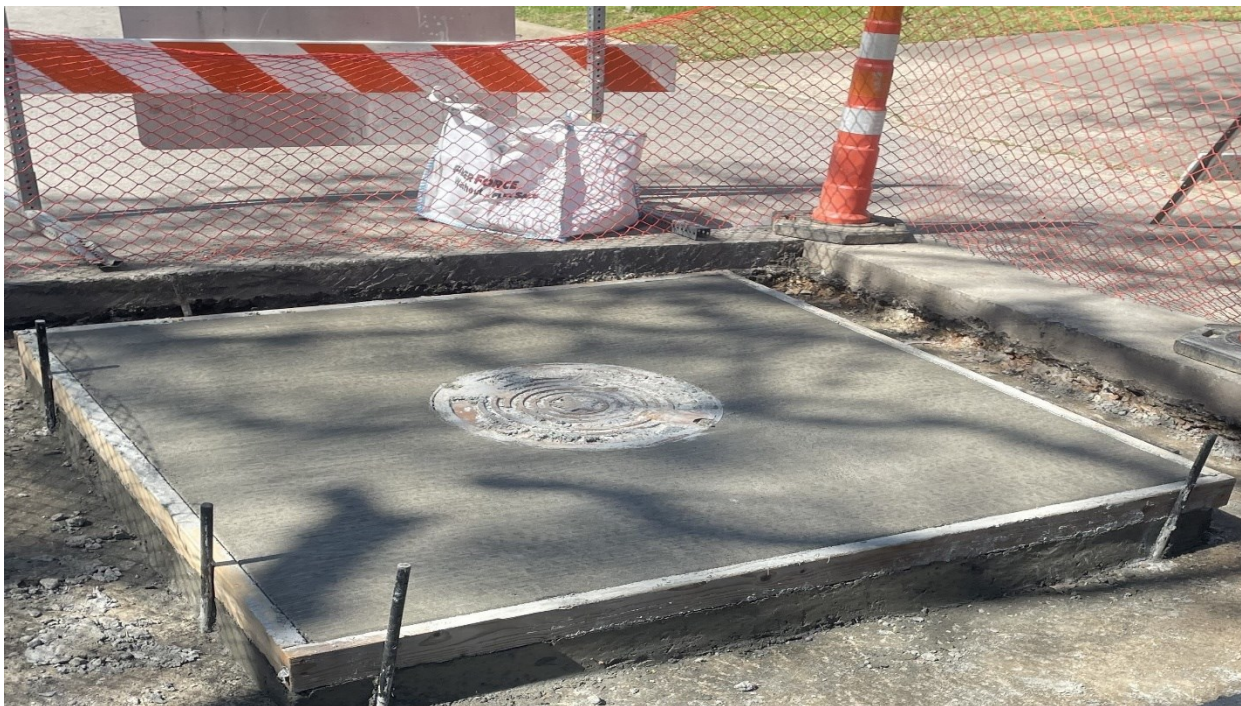
CONCRETE CAP FOR MANOLE PROTECTION
